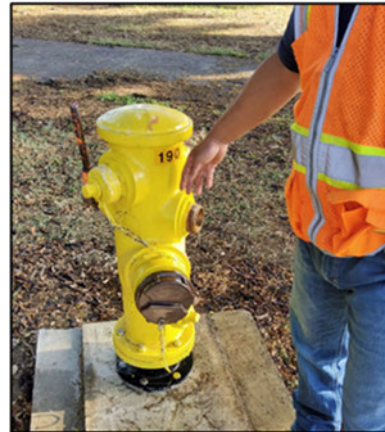
Figure 6-5 Leak Check
